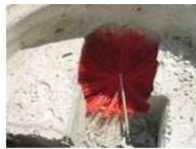
A 7" filter in a square septic tank baffle
