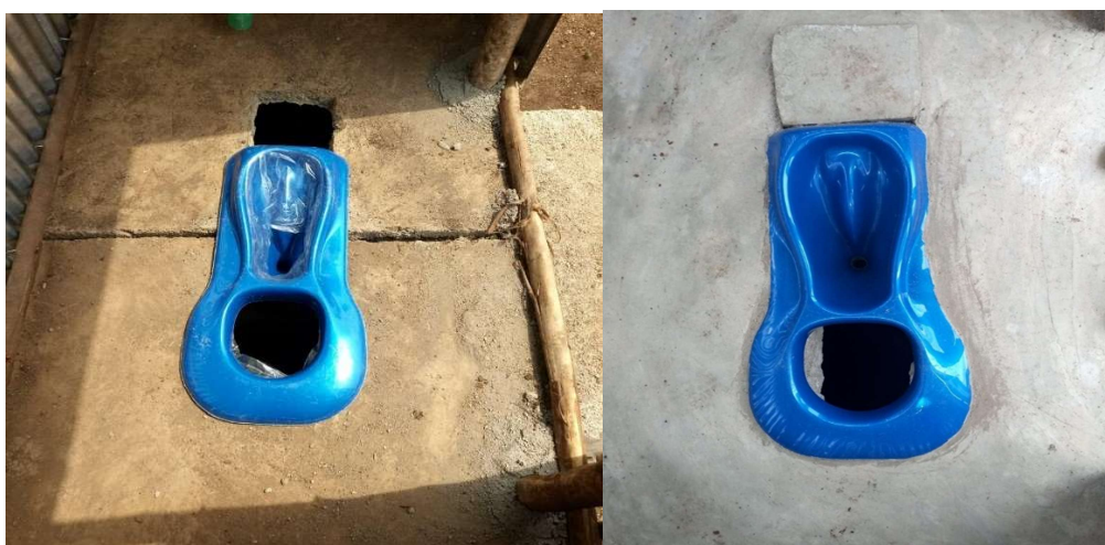
Fig 2: Squatplate inserted on finished concrete slab floor
