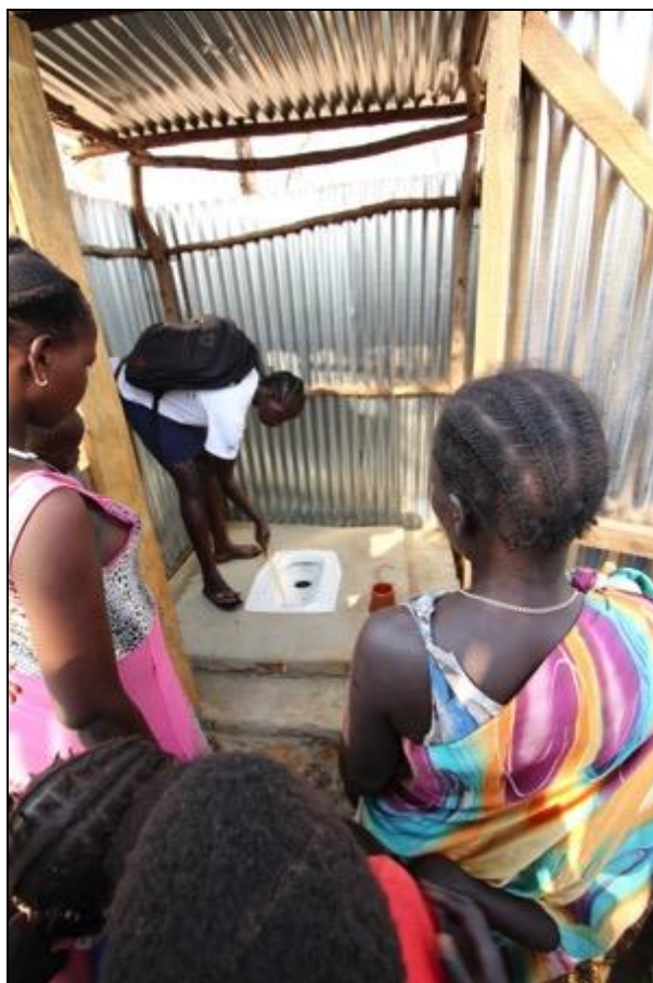
Figure 4. A demonstration of how to clean a Tiger Worm Toilet in Gambella.
