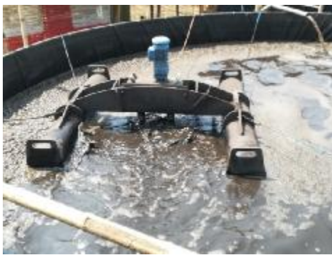
Surface mixing Unit
