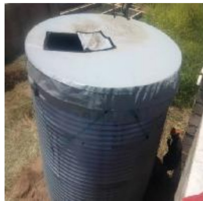
Top view of roofing
