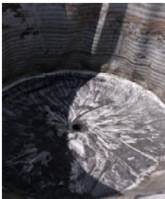
Outlet of tank
