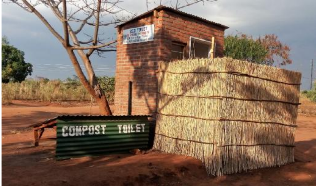
Earth Auger Toilets at Namisu Orphanage in Blantyre
