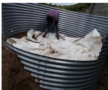
First level of metal sheets filled with sand
