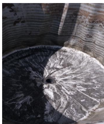
Outlet of tank
