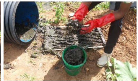
cleaning of bar screen
