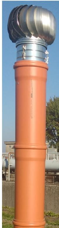
Figure 9 Ventilation: the top 2 segments of the infiltration shaft with fan mounted
