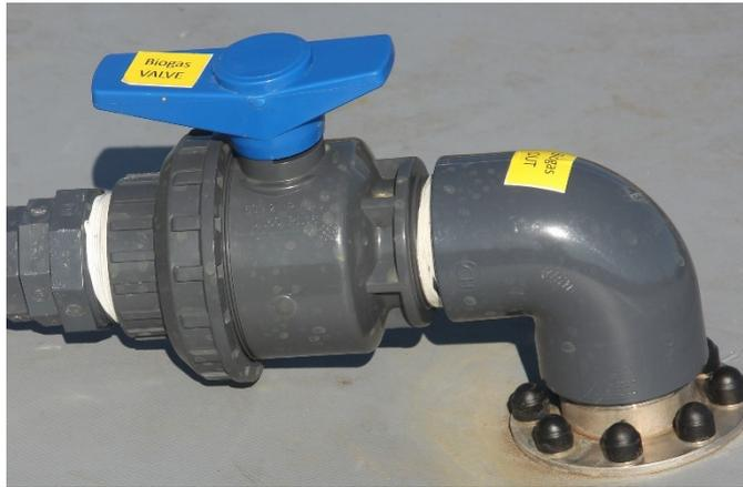
Figure 14 Gas valve open for initial filling
