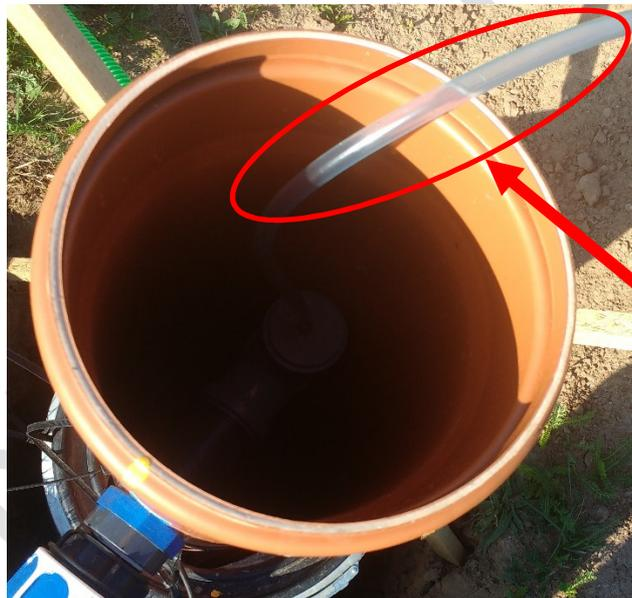
Figure 4 Tube leading up out of the second section of the infiltration unit
