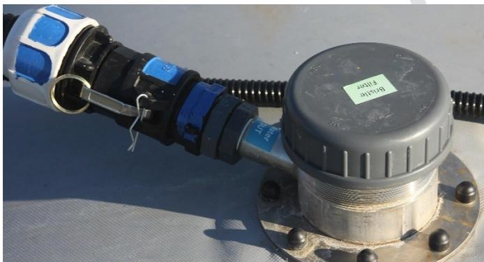
Figure 17 Wastewater discharge hose connection on the side of the tank
