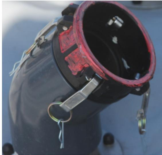
Figure 12 Wastewater intake connection
