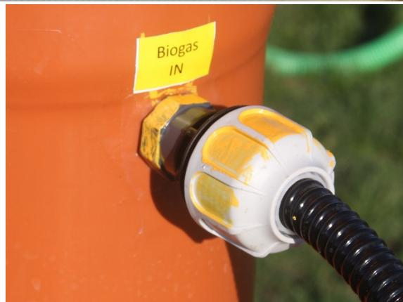
Figure 19 Biogas line connections (tank and filtration unit)
