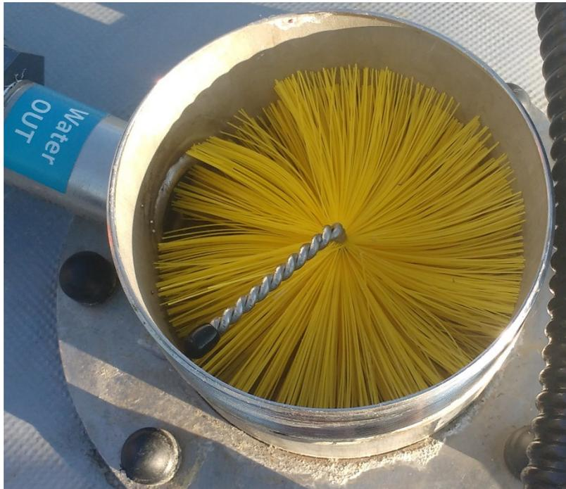
Figure 22 Installed bristle filter
