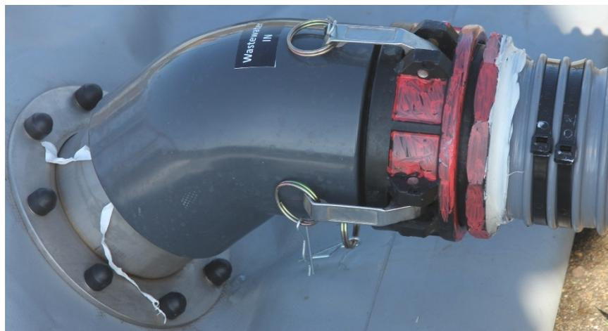
Figure 13 Inserted and locked wastewater intake hose
