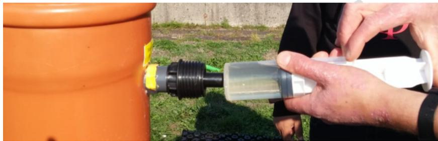
Figure 7 Filling the water trap
